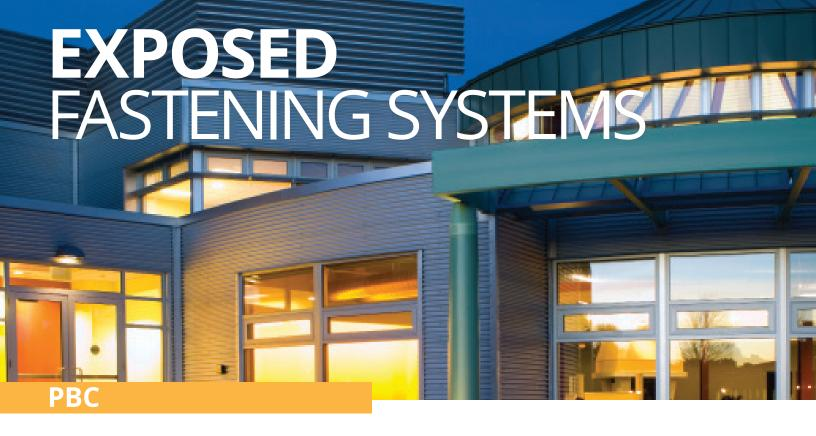
The PBC panels can be used for both roof and wall applications. PBC panels are attached to a building structure with exposed fasteners. The PBC panel is often used in horizontal applications on walls.
